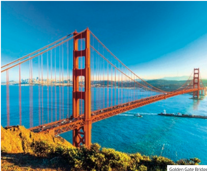
Golden Gate Bridge
