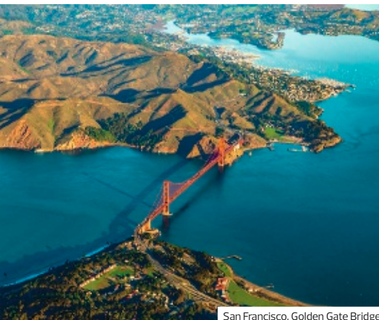
San Francisco, Golden Gate Bridge
