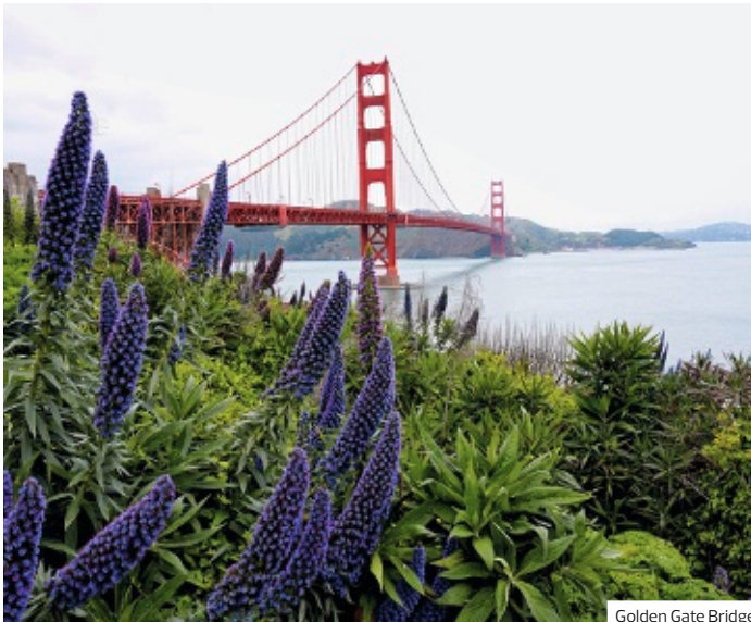
Golden Gate Bridge
