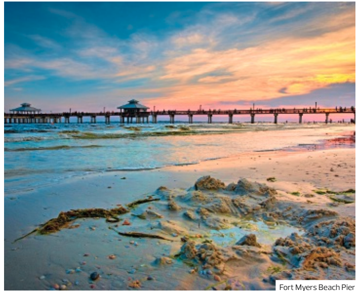
Fort Myers Beach Pier
